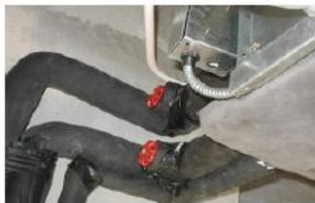
Equip valves at the inlet and outlet.
